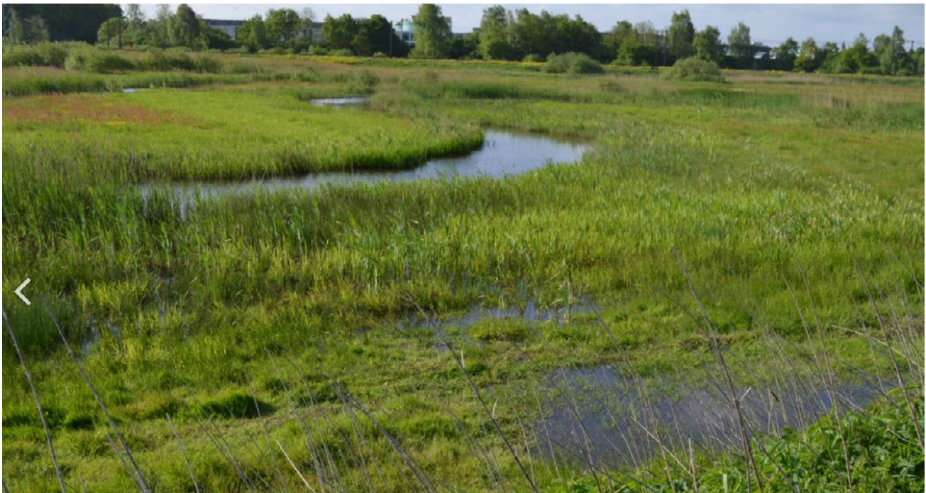
Constructed wetland of 7 hectares near Hooerveen, The Netherlands (source: ClimateScan )
