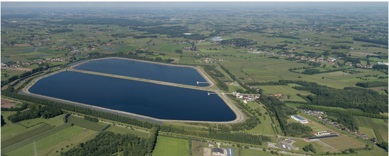
Aerial view on the water basins at Kluizen near Ghent for the collection of surface water for drinking water supply. © DE WATERGROEP
