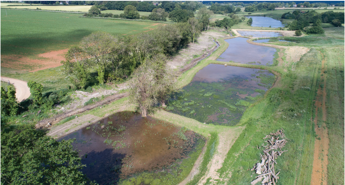
Aerial view of Ingodisthorpe recycling center with ponds forming the new treatment wetland © ANGLIAN WATER
