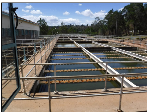
Plate 5: Chebara Treatment Works
