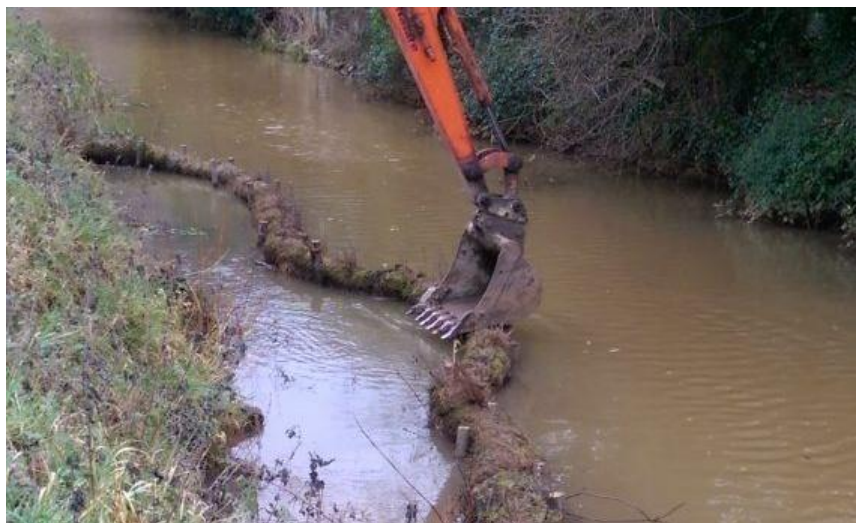
Berm creation with coir rolls | River Gaywood, Norfolk. ©Norfolk Rivers Trust
