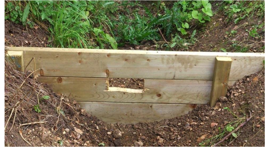
Leaky dam in ditch | Upper River Nar, Norfolk. ©Norfolk Rivers Trust
