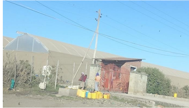
Figure 14 Water access point in the upper catchment of the Dire Dam
