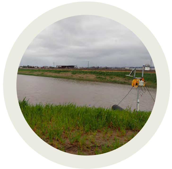
A recharge basin in the Pajaro Valley. © Andy Fisher
